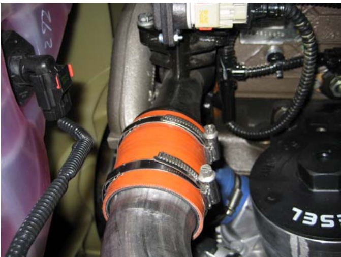
Figure 6 Installation of Mixer Pipe Hose Clamps
