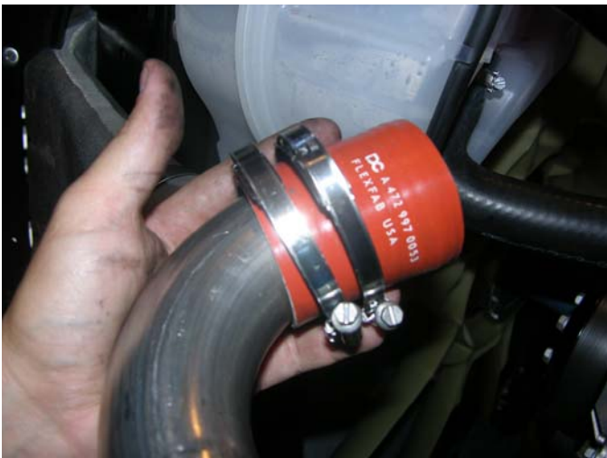
Figure 4 Installation of Mixer Pipe Hose and Clamps
